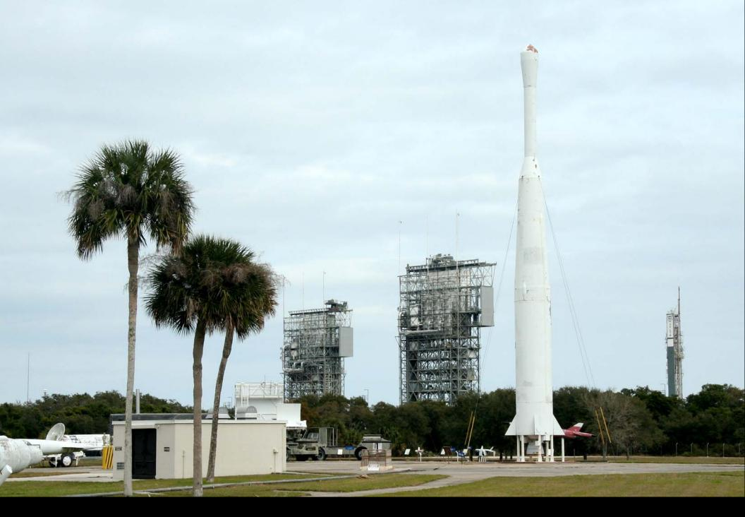
The Launch Control was in a blockhouse only about 400 feet / 120 m from the rocket to keep analog cable lengths short for reliability.
