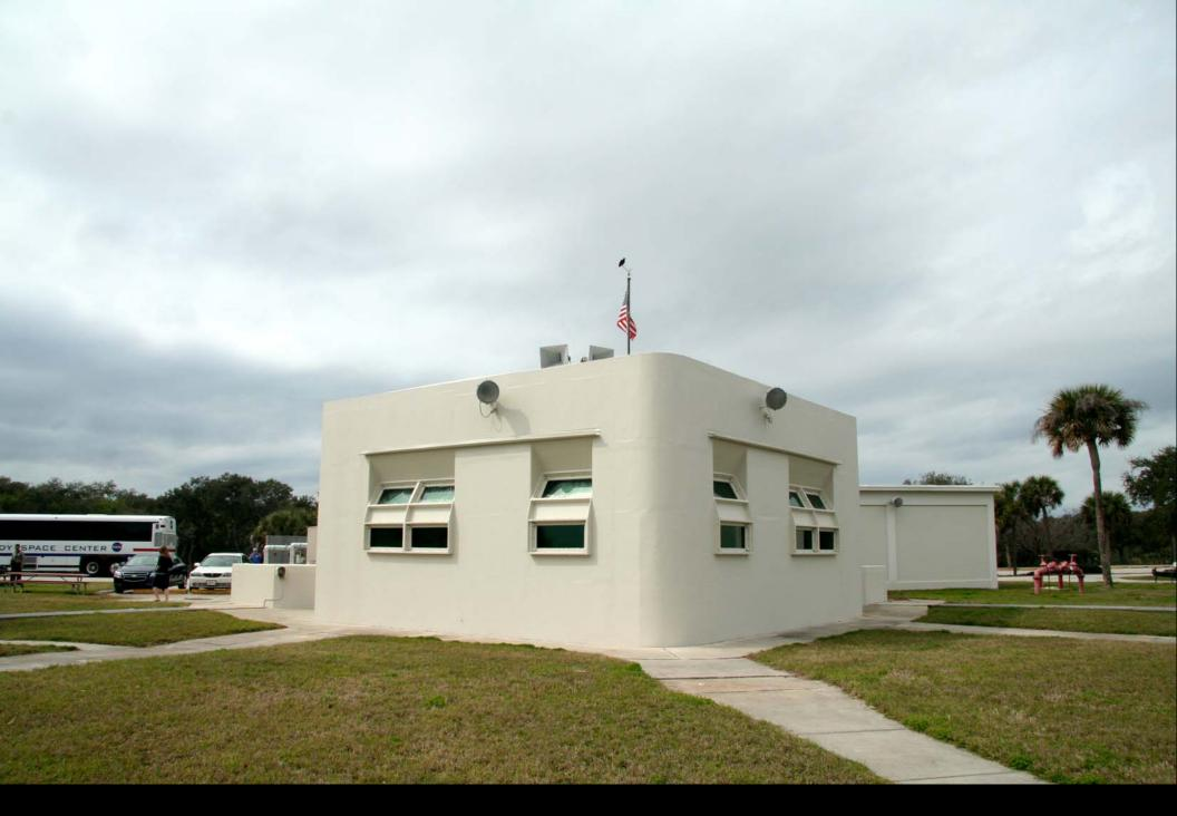
Block houses had concrete walls that started at2 feet thick and got much thicker as more dangerous rockets were developed.
