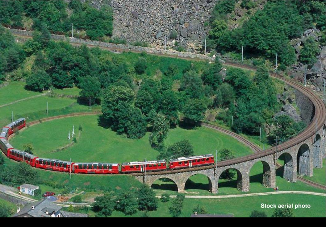
The Circular Viaduct in Brusio accomplishes an elevation change of 66 feet on the spot.
